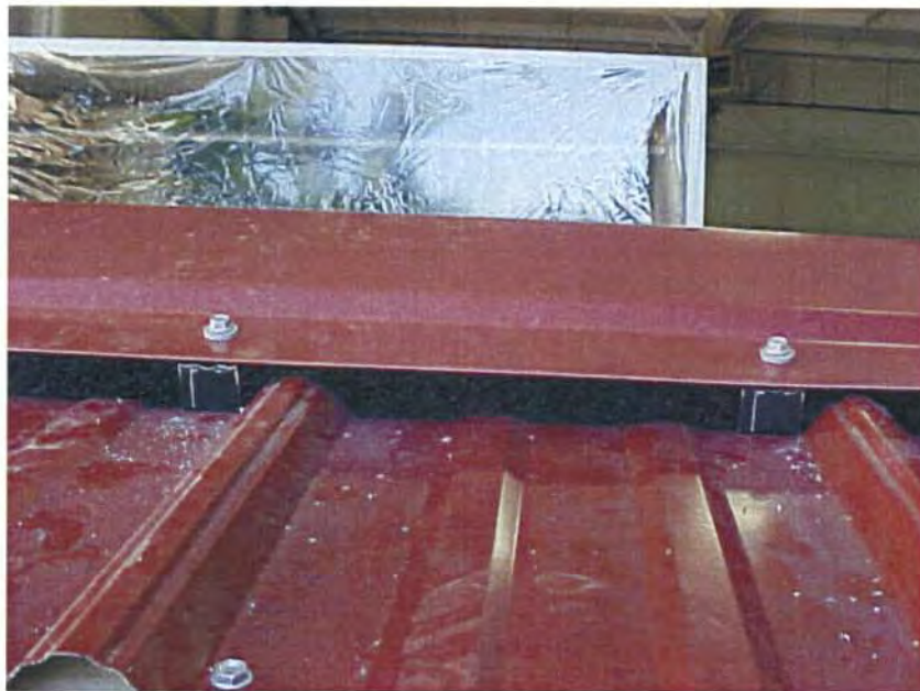
Photo No. 4 Ridge Cap Installed onto Clips
