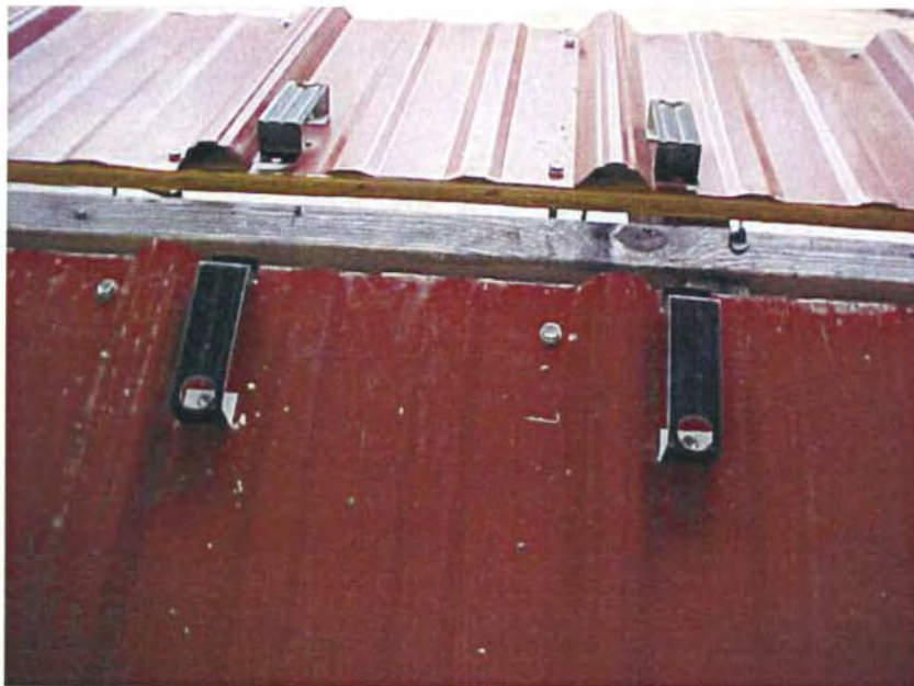
Photo No. 2 Clips Installed at the Ridge
