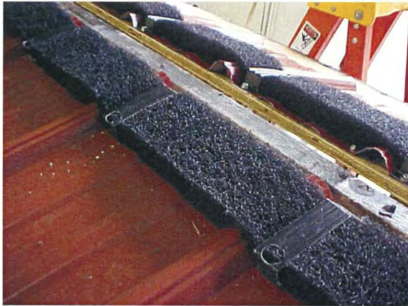
Photo No. 3 Vent Material Installed under Clip
